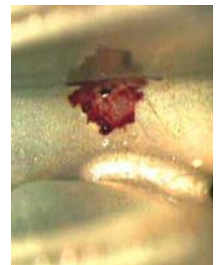
Figure 8.30 (b) Pitting corrosion in stainless steel 316.
