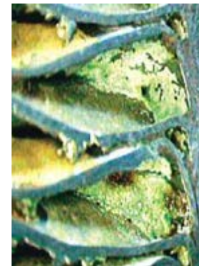
Figure 8.30 (a) General copper corrosion.
